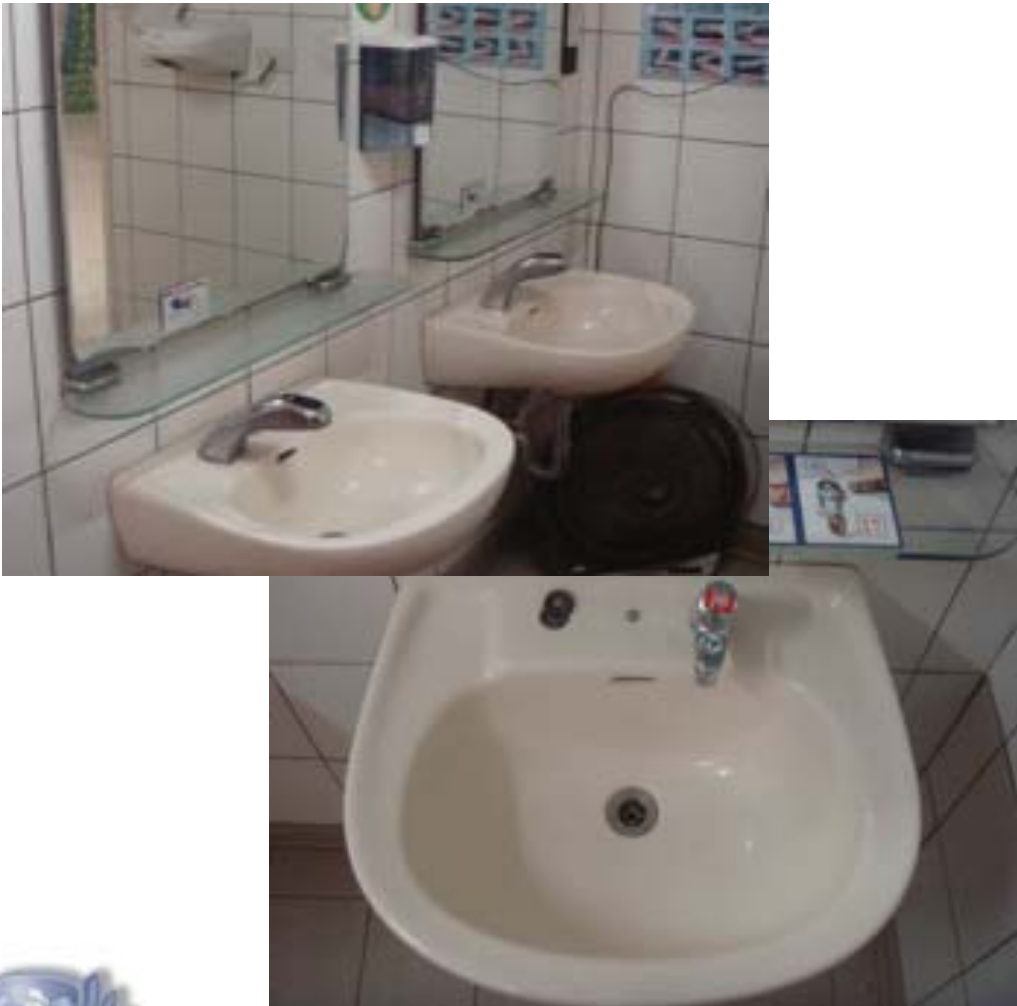
electronic sensor water taps
