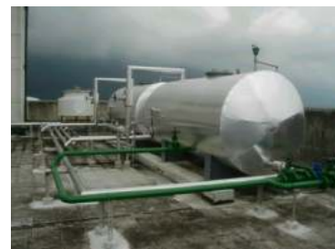
Buddhist Dalin Tzu Chi General Hospital- Heat pump system
