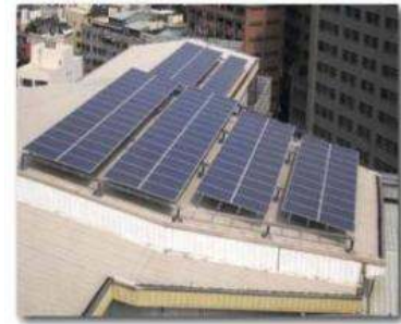
Changhua Christian Hospital- Photovoltaic system
