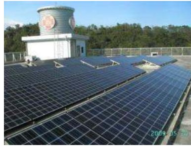
Mackay Memorial Hospital Taitung Branch- Photovoltaic system
