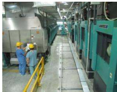
Chang-Gung Memorial Hospital Taoyuan Branch- Tunnel washers
