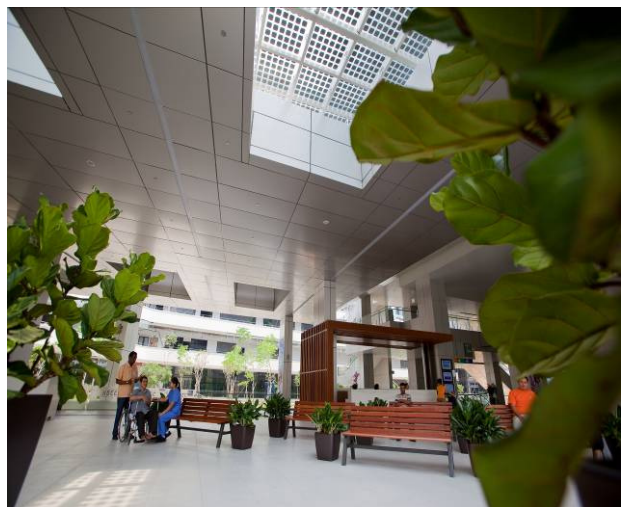
Alexandra Health Cluster- Main Lobby with solar panels visible
