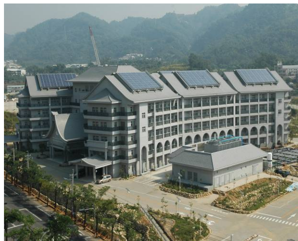
Buddhist Taichung Tzu Chi General Hospital- Photovoltaic system
